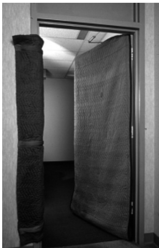
Unique door protection devices minimise risk of damage to the office and furniture.
